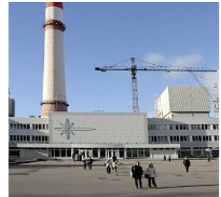
The Leningrad plant is in the closed city of Sosnovy Bar near to Saint Petersburg
